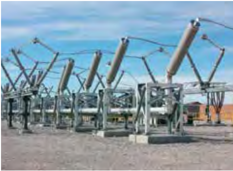
Power Transmission and Distribution
