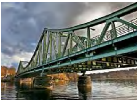
Bridge and Highway
