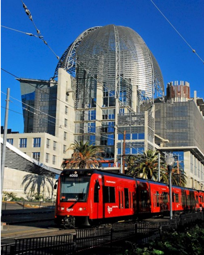
The San Diego Central Library façade and dome utilizes hot-dip galvanized hot-rolled sections, plate, and hollow structural steel sections.
