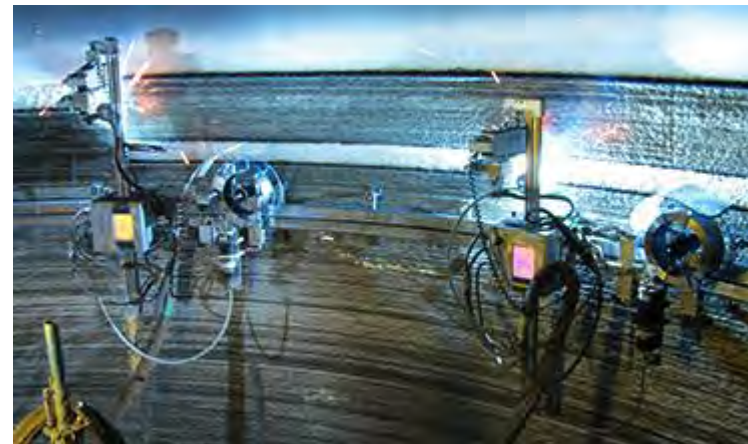
Coke Drum Repair
