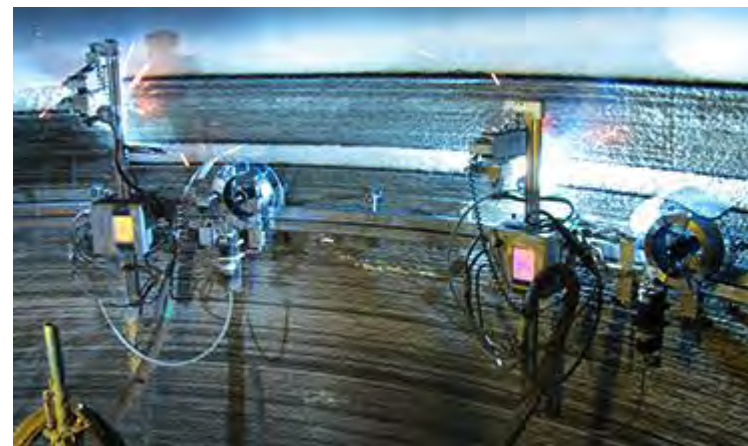
Coke Drum Repair
